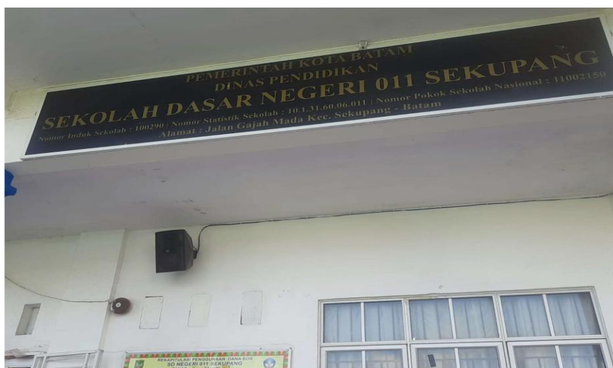
Figure 1. Main Building of SD Negeri 011 Sekupang Batam ,May 2026.
