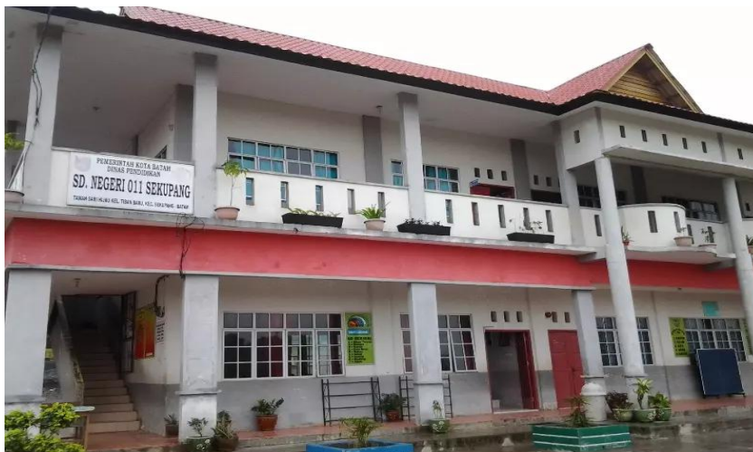
Figure 2. One of the main buildings of SD Negeri 011 Batam, May 2026
